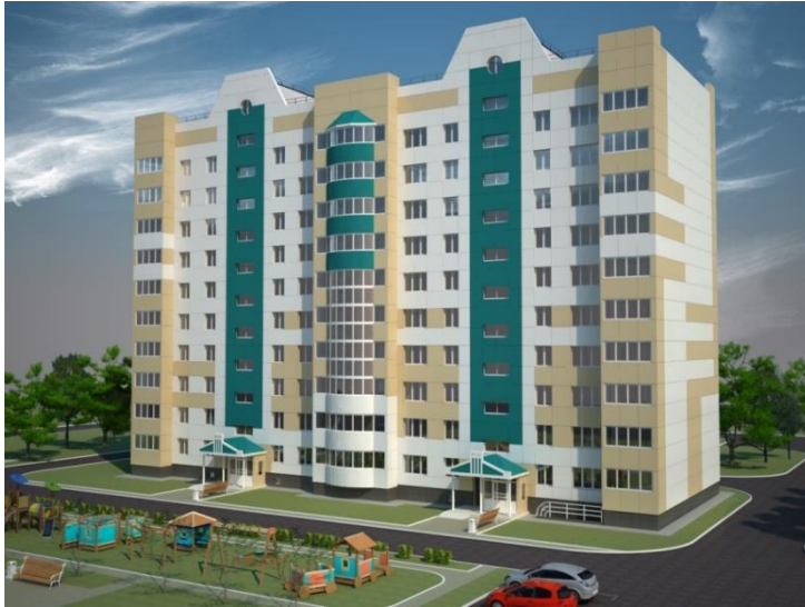
Figure 11. Large-panel buildings series KPD-330E (Customer Success story Autodesk 2014)
