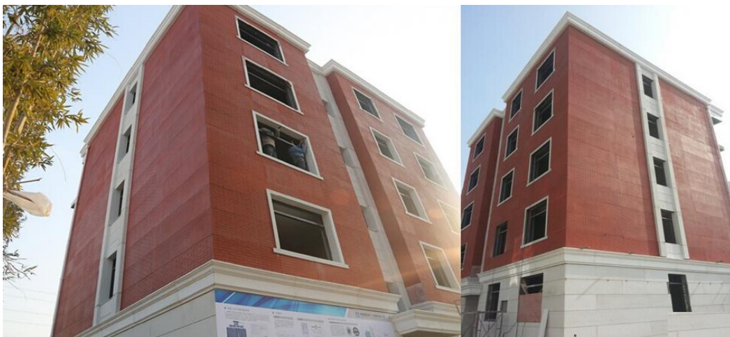
Figure 18.a. A 6-story tall building which has been 3D printed by Winsun (3D print Website)
