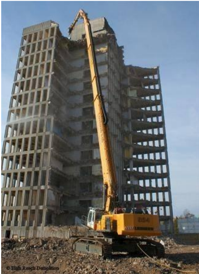
Figure 1.2 High reach arm excavator
