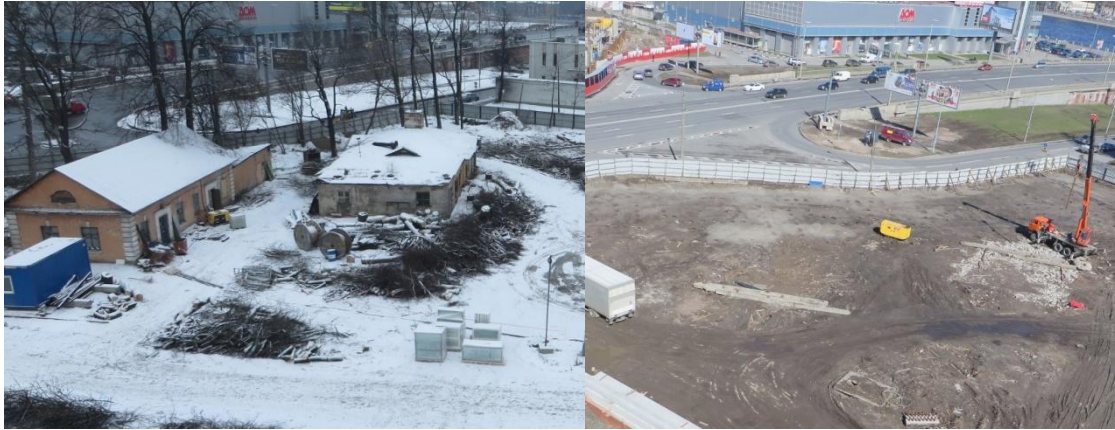
Figure 5.1 Skandi Klubb Construction site before and after demolition.
