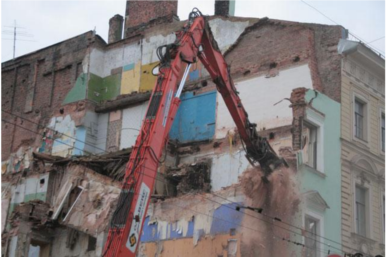
Figure 4.1 Demolition in the city center
