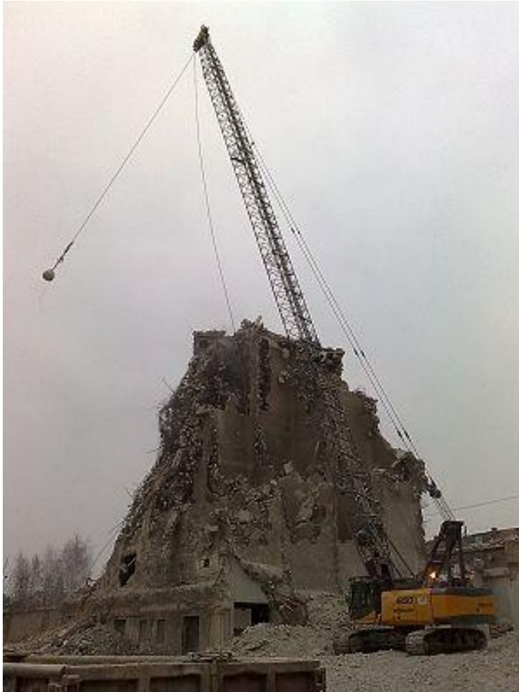
Figure 2.1 Demolition with wrecking ball
