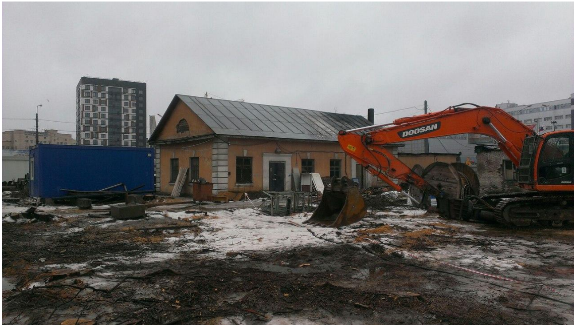
Figure 5.2 Demolition equipment on Skandi Klubb
