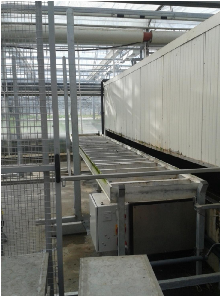
FIGURE 3. Push-in position P8 (Fedotova 29.03.2016)
