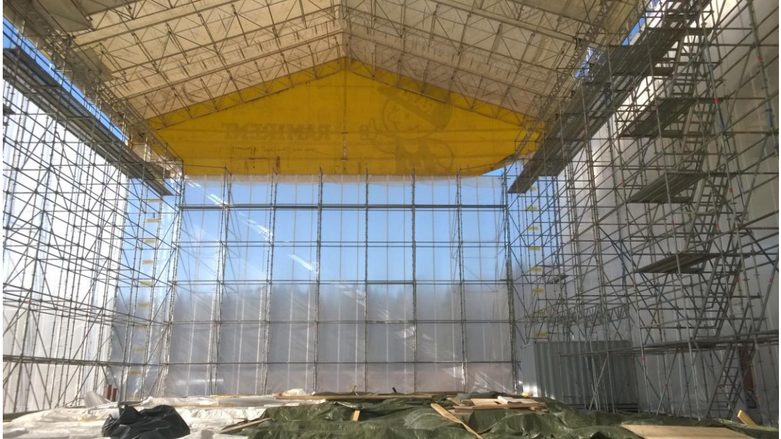
Figure 3. Inside of the finished Keder weather cover system.
