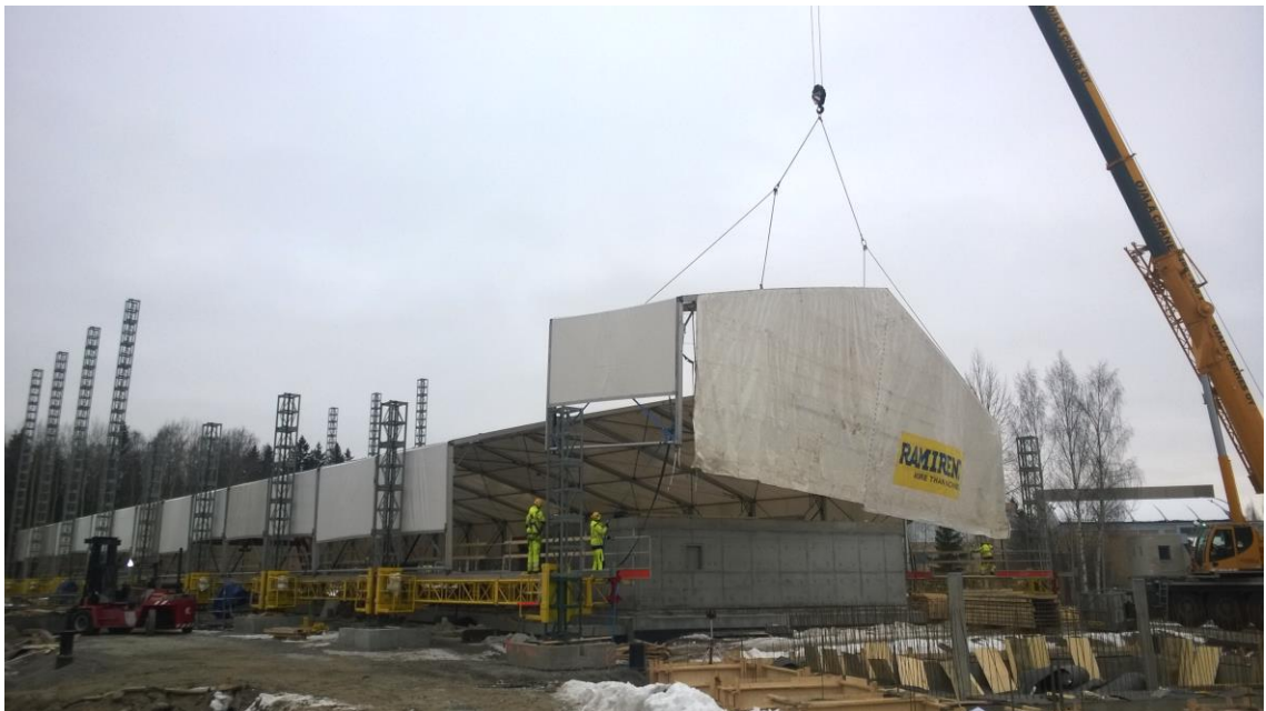
Figure 5. Last one of the roof modules being lowered to its place.
