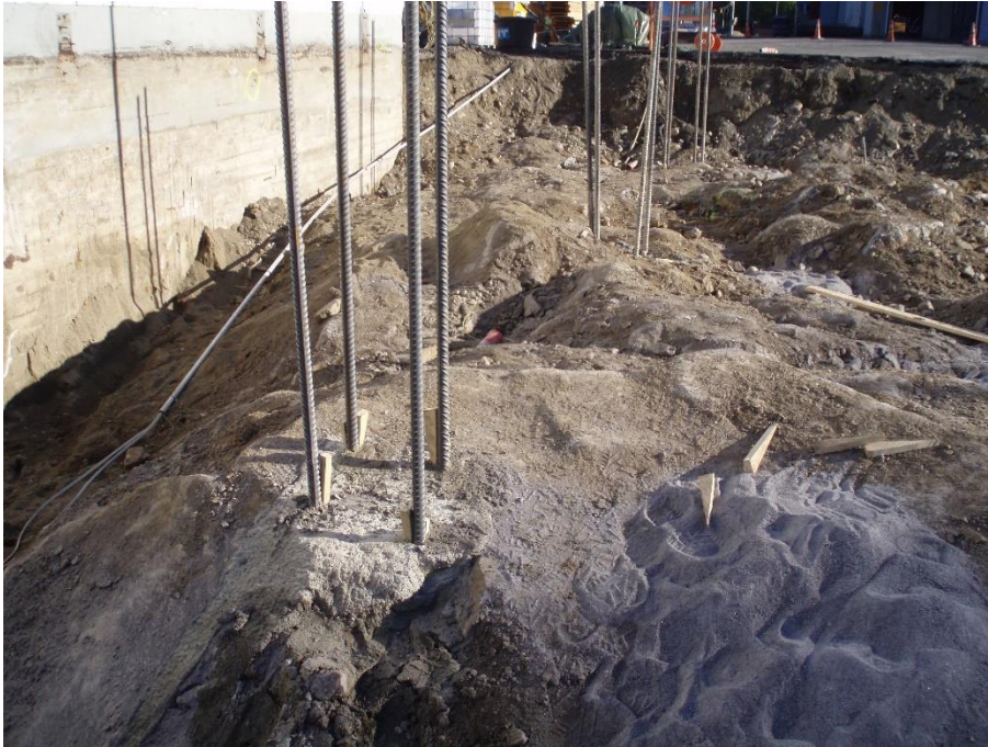
Figure 6, Steel anchors glued in the bedrock, photo by Hannele Kulmala
