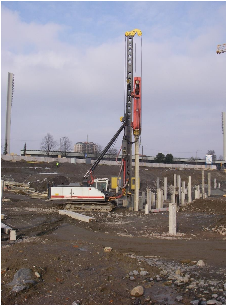
Figure 5, Concrete pile foundation, photo taken by Hannele Kulmala
