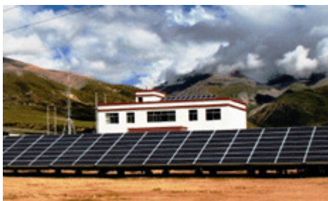
demonstration power plant
