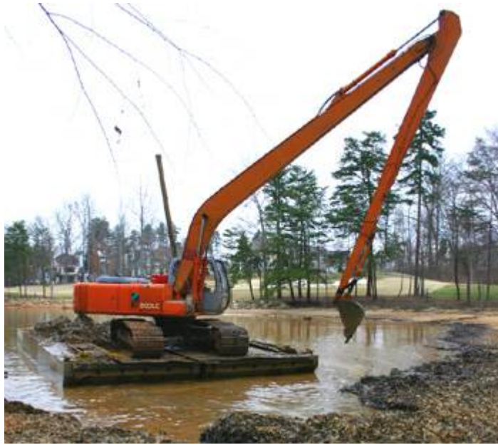
FIGURE 4. Excavator dredging (Lakeside Marine Construction, 2008)
