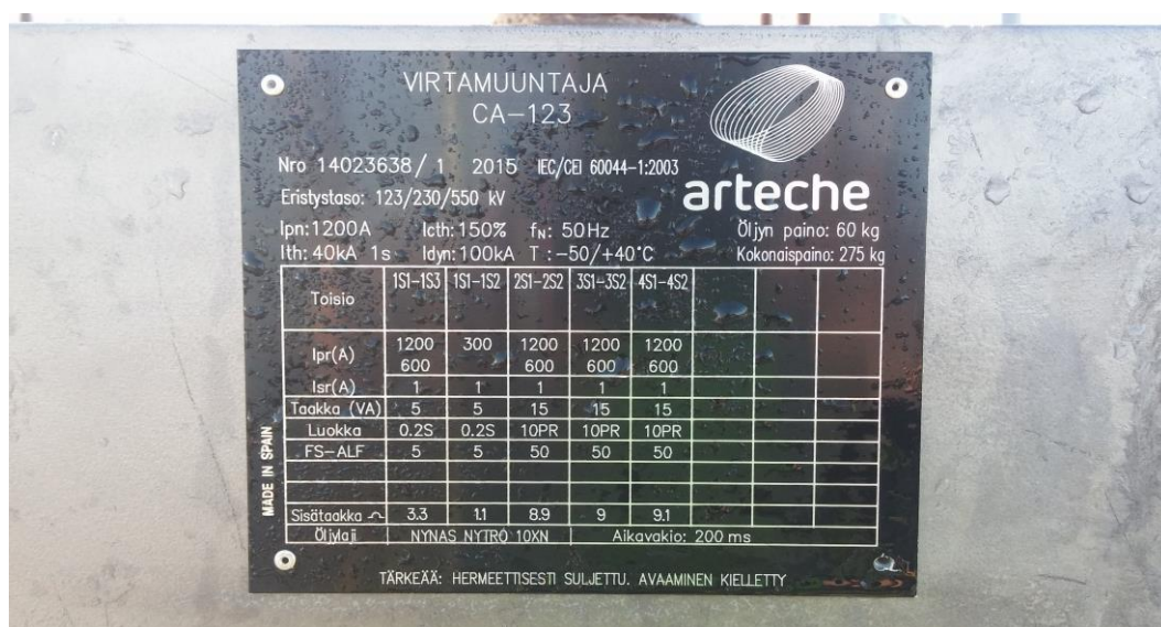
Figure 8. 110 kV Current Transformer
