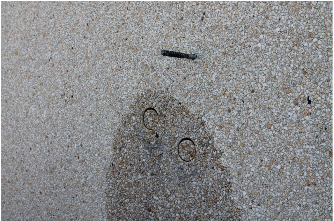
Picture 3. The result of drilling.
