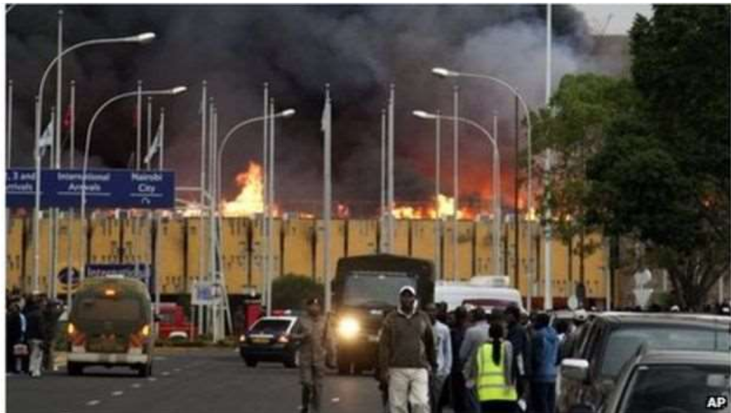
Figure 2. The fire at JKIA 2013
