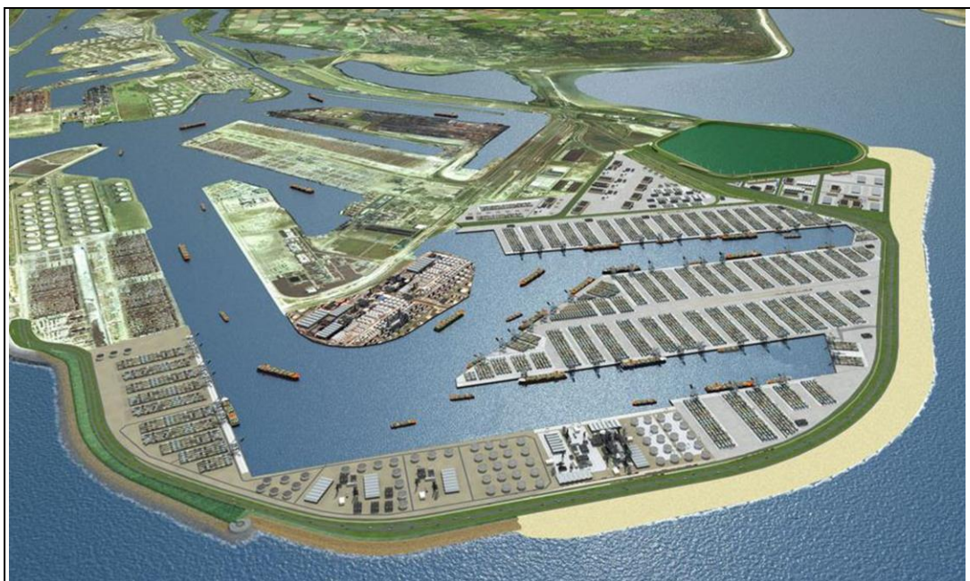
Picture 4. Rotterdam Multimodal Container Terminal. (Website of Dredging Today 2016)
