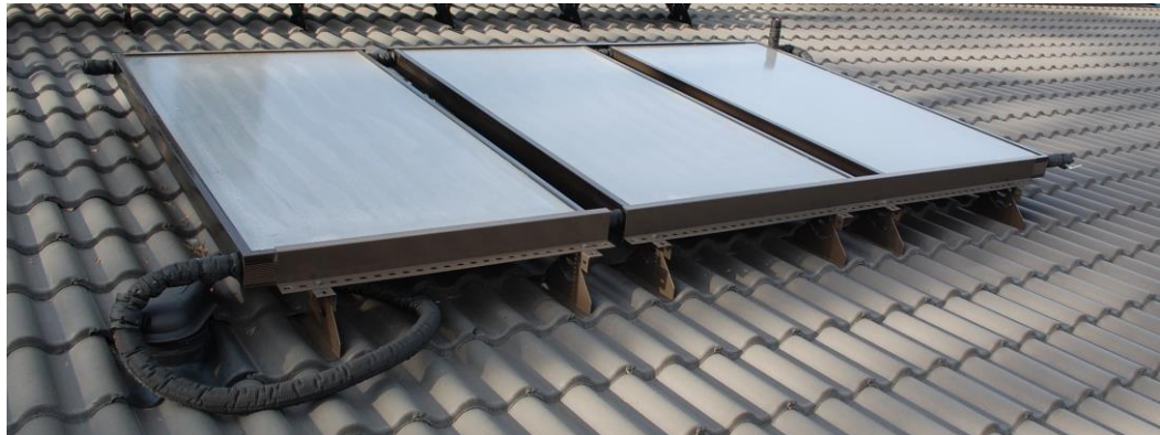
Figure 5. Heat pipe system with a cover
