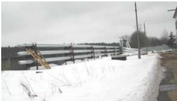
FIGURE 16. The heat exchanger used in sewage-source heat pump system in Zelenograd, Russia /30/
