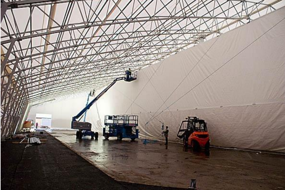
FIGURE 6. Installing inner fabric (BESTHALL PROCEDURE 2012, 38)
