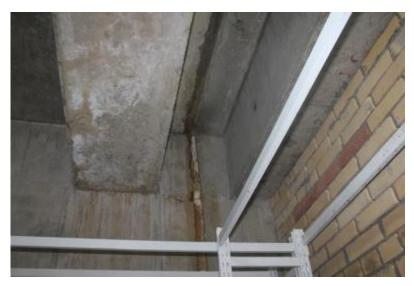
Figure 26. Deformation joints
