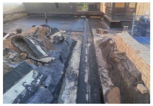
Figure 34. Removing of roof covering
