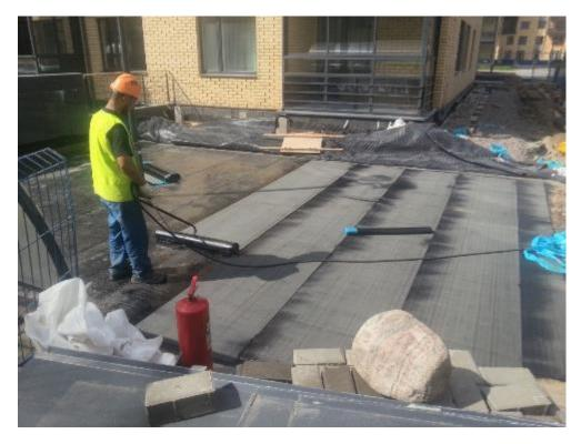
Figure 35. Roof waterproofing with Ultranap membrane slope (1:70)
