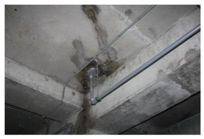
Figure 25. Water filtration through drainage system
