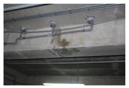
Figure 24. Water filtration through drainage system
