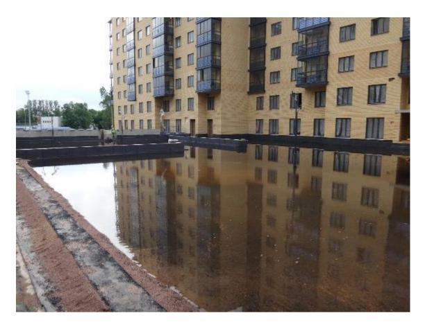
Figure 42. Waterproofing testing
