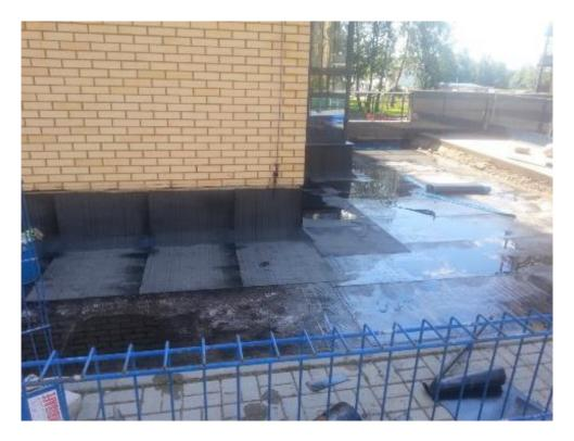
Figure 36. Building walls waterproofing with Icopal H
