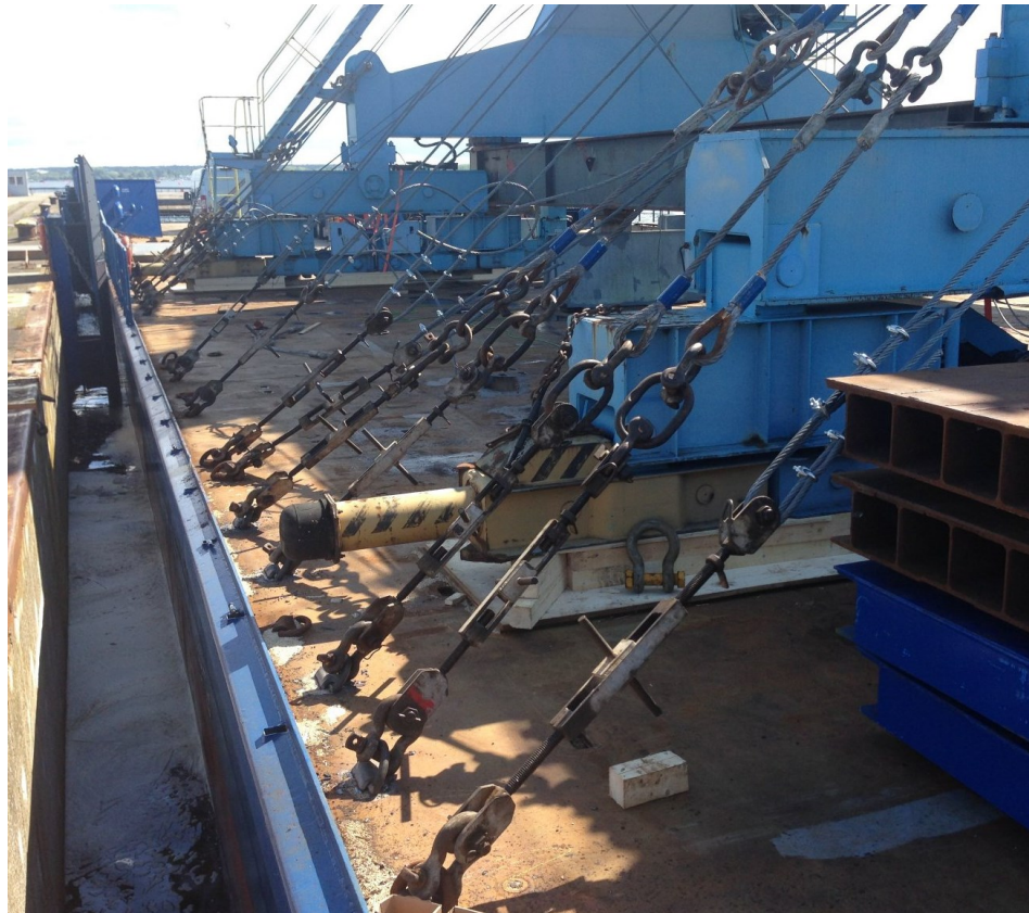
Figure 8 Cargo securing equipment in use ( www.craftmer.fi )
