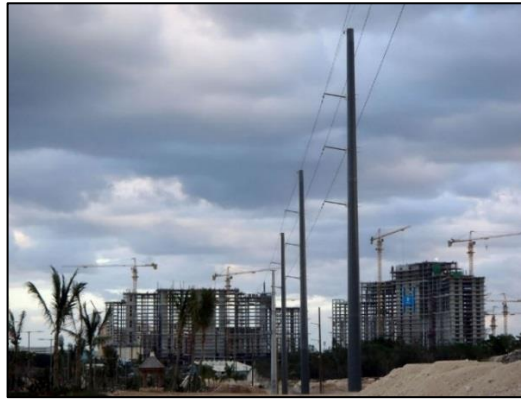
Figure 22. Vertical HV single line assembly.
