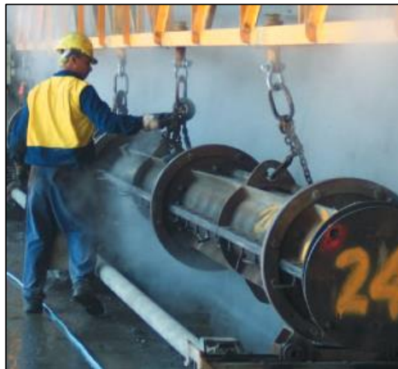
Figure 17. Manufacturing of spun concrete pole. /27/
