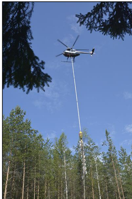
Figure 33. Helicopter trimming for line passage in action. /40/
