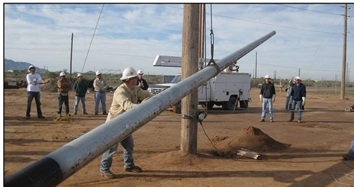
Figure 18. Steel pole erection. /28/
