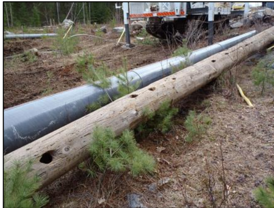
Figure 16. Wooden pole is replaced with composite pole. /25/
