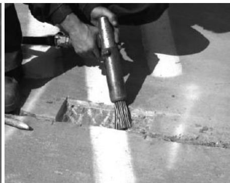
Figure 3. Removal of concrete.
