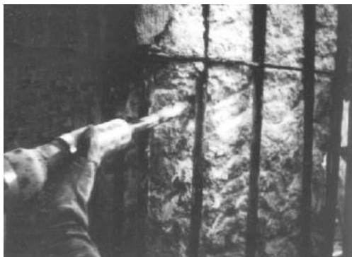
Figure 2. Removal of concrete.
