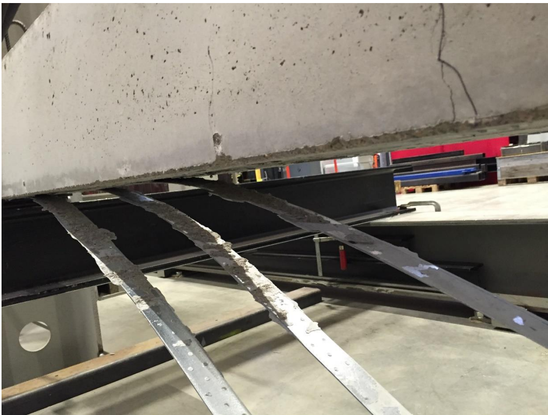
Partially reinforced beam failure mode
