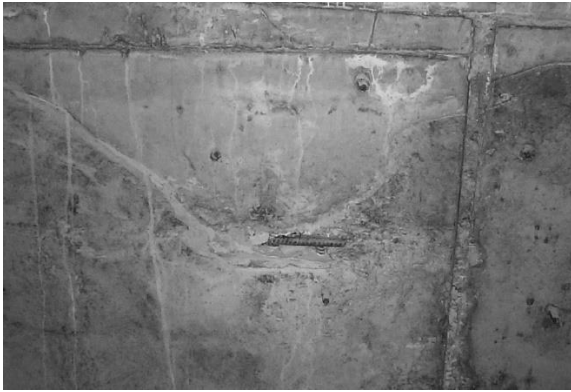
Exposed rebar
