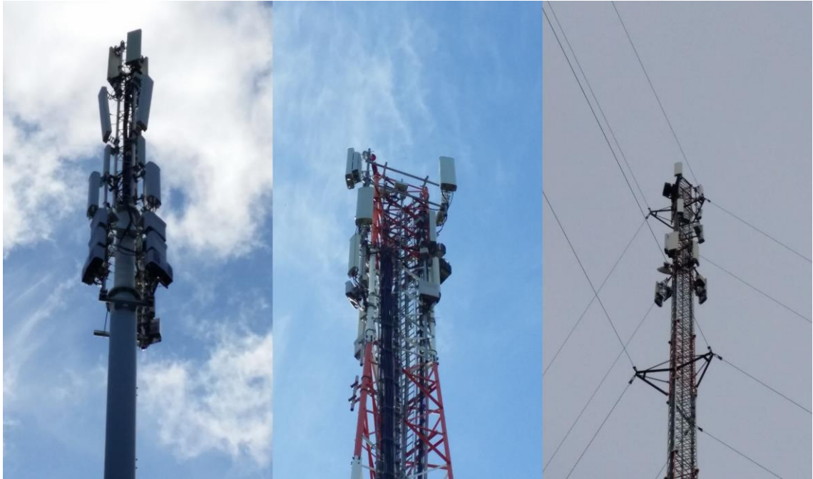
Figure 4. (a) Tubular steel mast 25m (b) Free-standing reinforced steel 40m (c) Supported reinforced steel 80m
