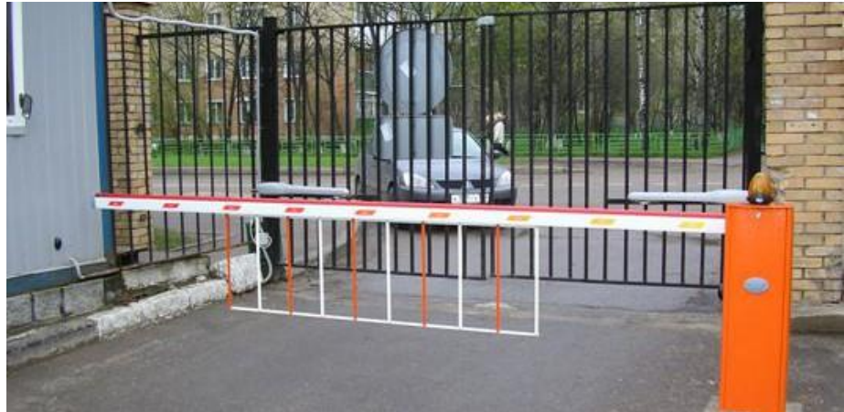
FIGURE 2. Automatic gates. (Oleg Chirkov, 2008)
