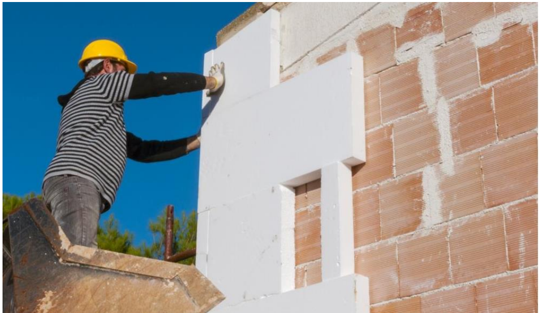
IMAGE 2. Insulation plates being applied in construction (WA Polystyrene 2017b)
