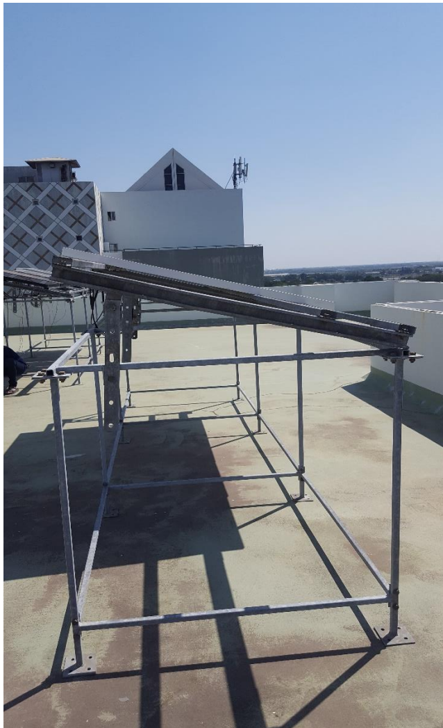
Figure 4. Finished rack for the solar panels
