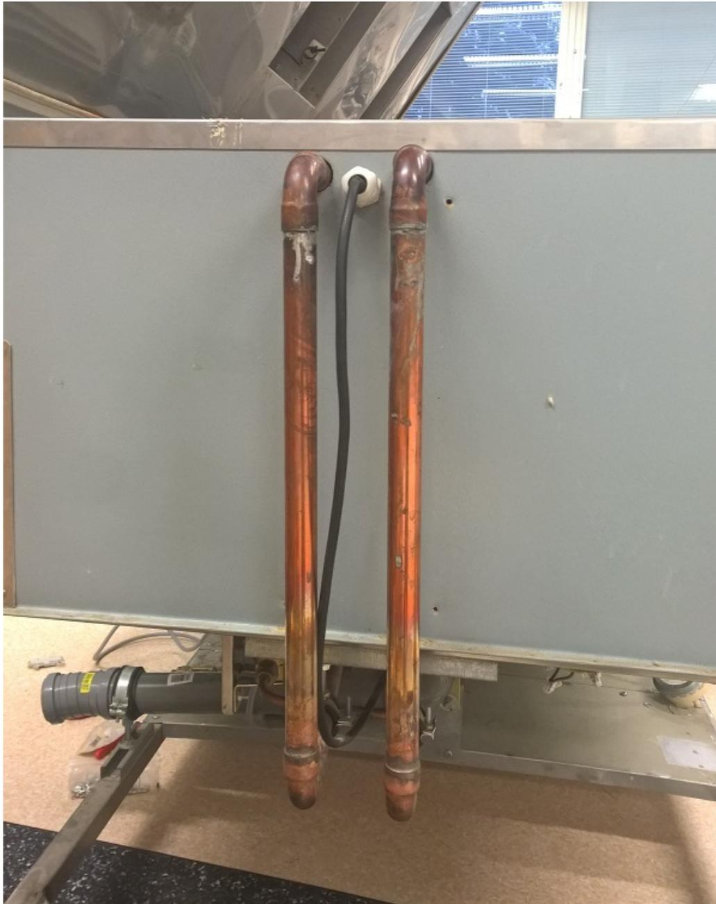
Figure 11. Hot inlet water pipe and overflow pipe looks from the outside (photograph taken by the author)
