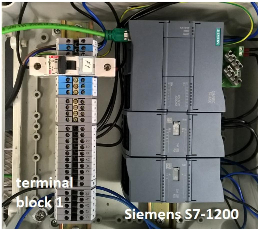
Figure 4. Terminal block 1 and PLC controller (photograph taken by the author)
