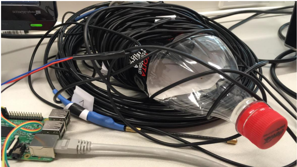
Picture 4. Dallas temperature sensors cable.
