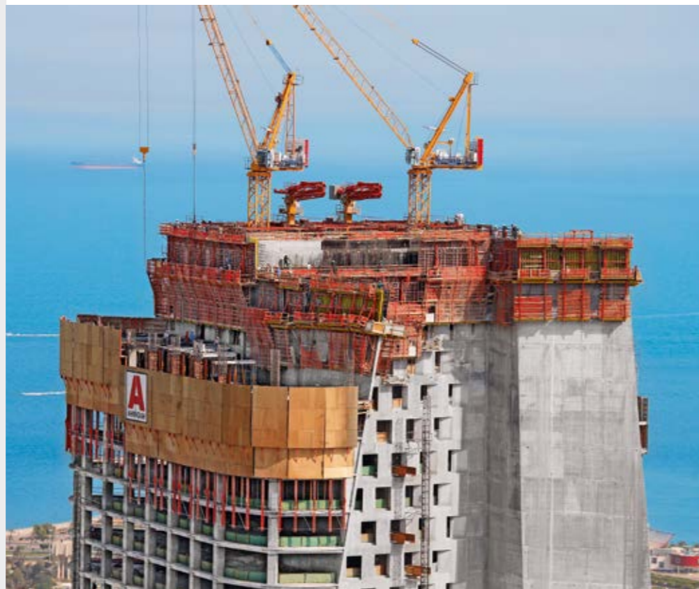
Picture source: PERI GmbH, Weissenhorn
