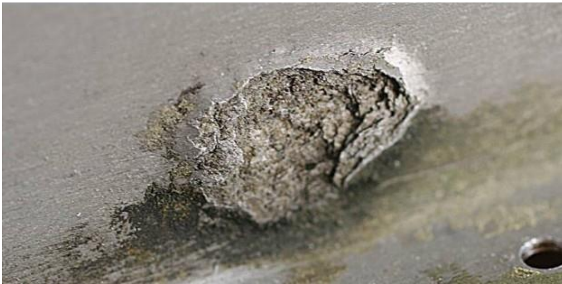
PICTURE 2. Intergranular corrosion (DVI Aviation n.d)
