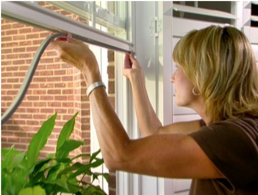
FIGURE 1. Weatherstrip installation (Adapted from Monzon Sarah 2014.)
