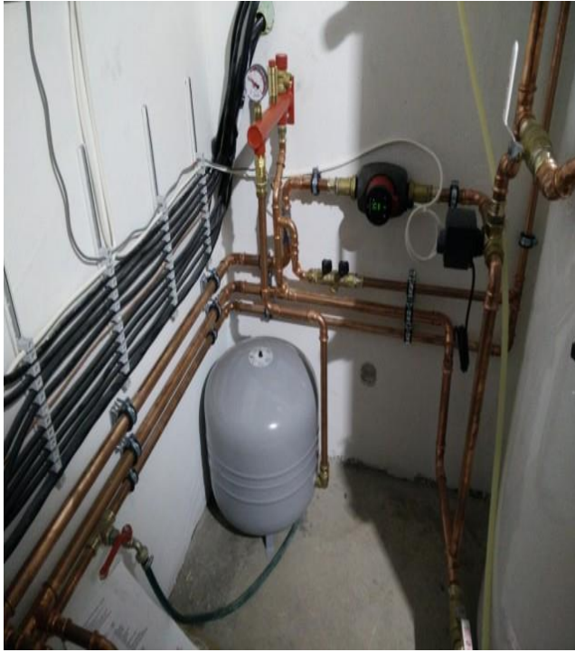
Figure 7. Pump used for the circulation of hot water for ground-floor
