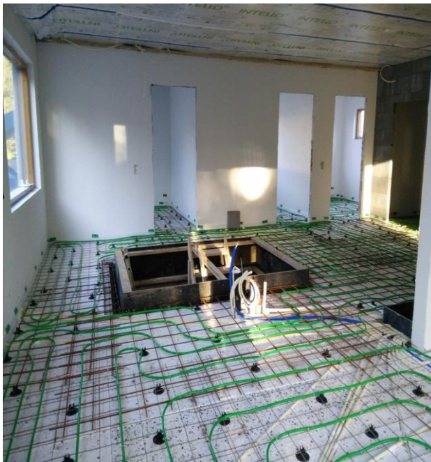
Figure 5. Underfloor heating pipe installation
