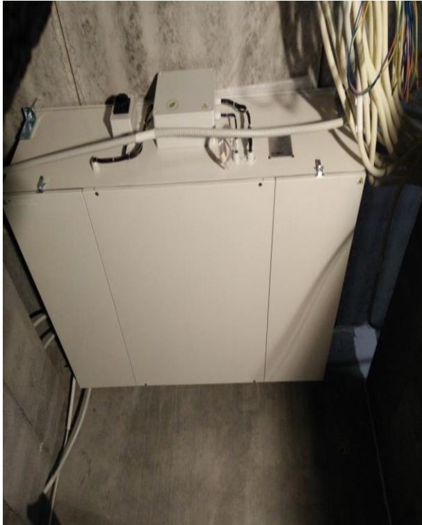
Figure 2. PAUL heat recovery system which is placed in ground floor
