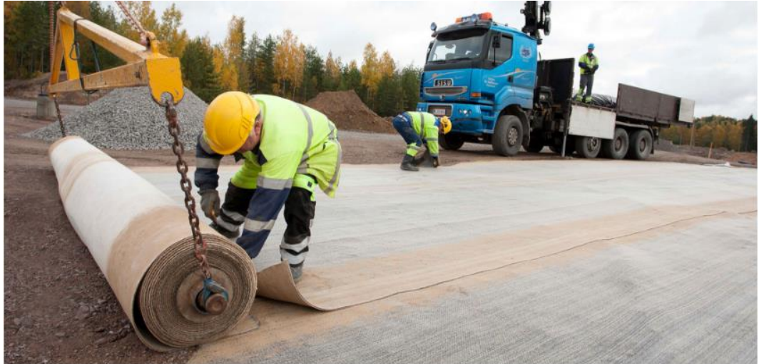
IMAGE 8. Bentonite clay liner being assembled for groundwater protection in highway construction site. (Kaitos Oy 2017)
