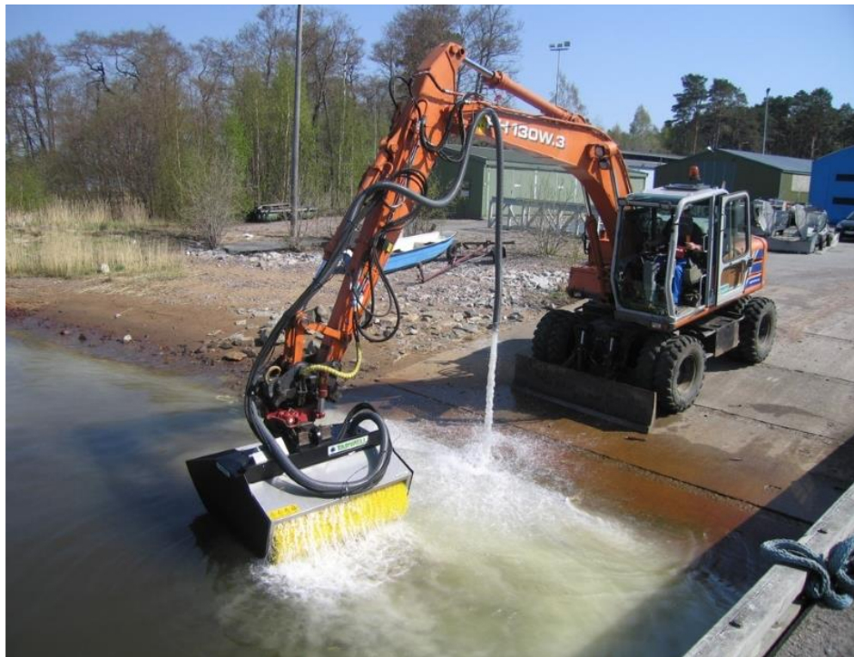
IMAGE 5. A brush skimmer installed on an excavator. (Saarioinen 2016)
