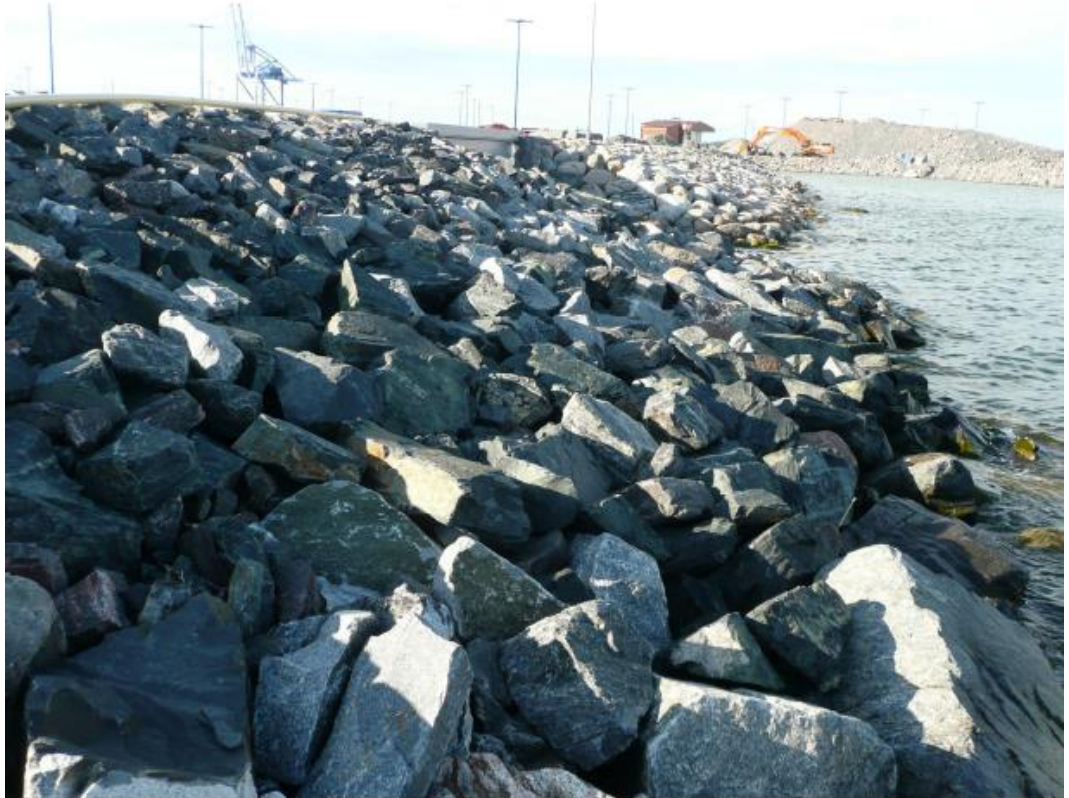
IMAGE 7. An example of heavy erosion protection on a manmade shore embankment at Vuosaari harbour in Helsinki. (Finnish Consulting Group 2017)
