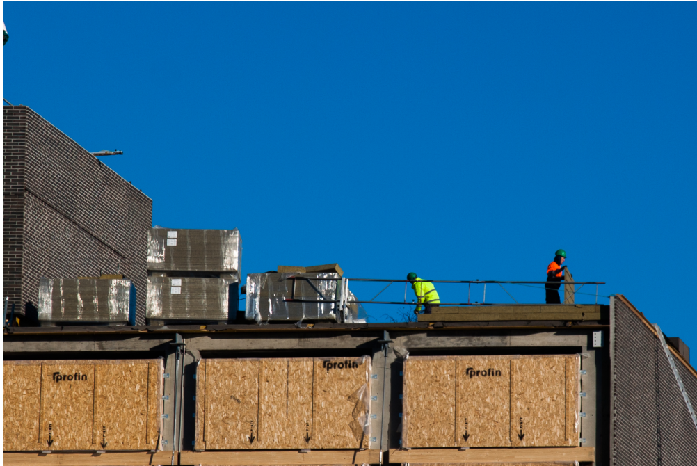
Figure 5, Builders working in Kruunuvuorenranta, Helsinki.
