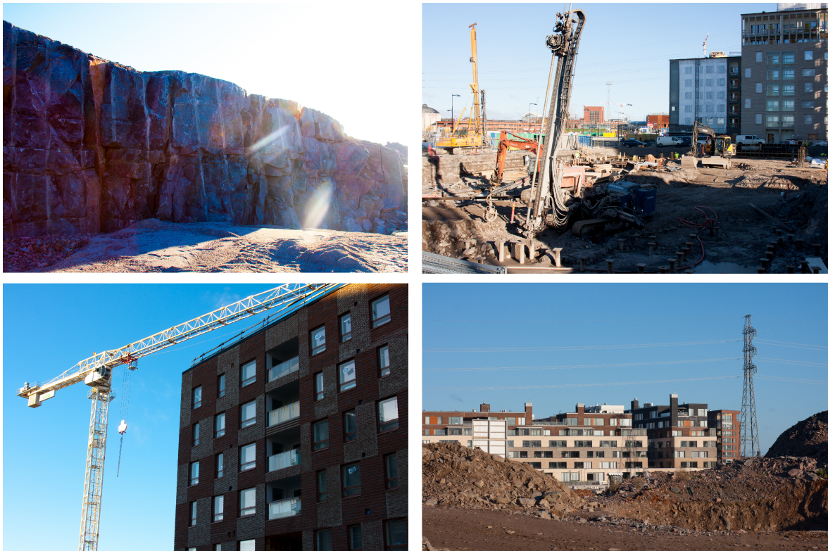
Figure 7, Construction stages in building site, Kalasatama, Helsinki.
