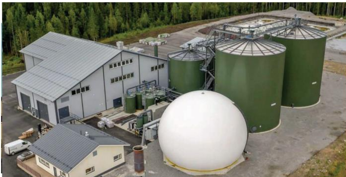
FIGURE 32. Kuopio Biogas plant
