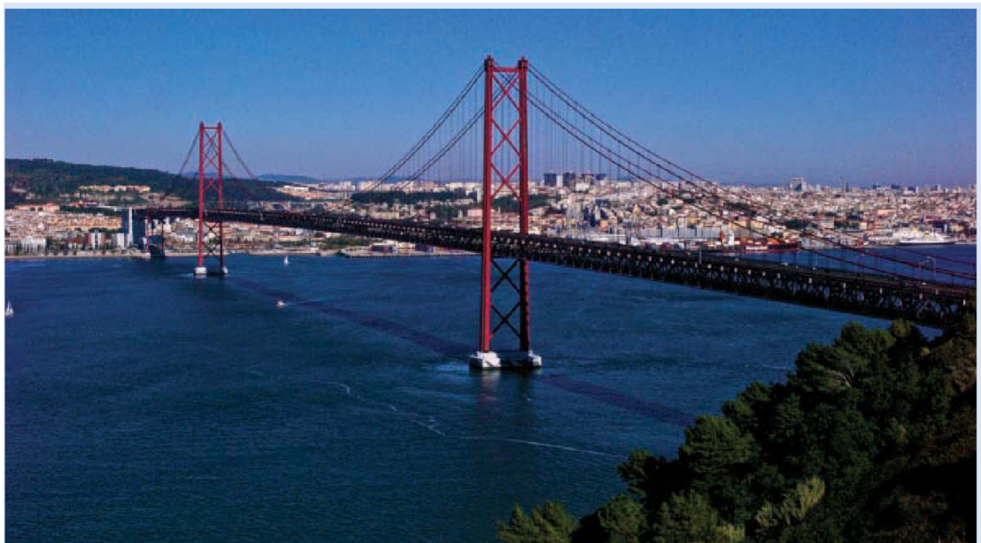
Figure 4. A bridge crossing Tagus river in Lisbon, Portugal [5]
