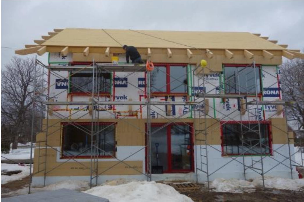
Figure 9. Half-way finished wall insulation [42].
