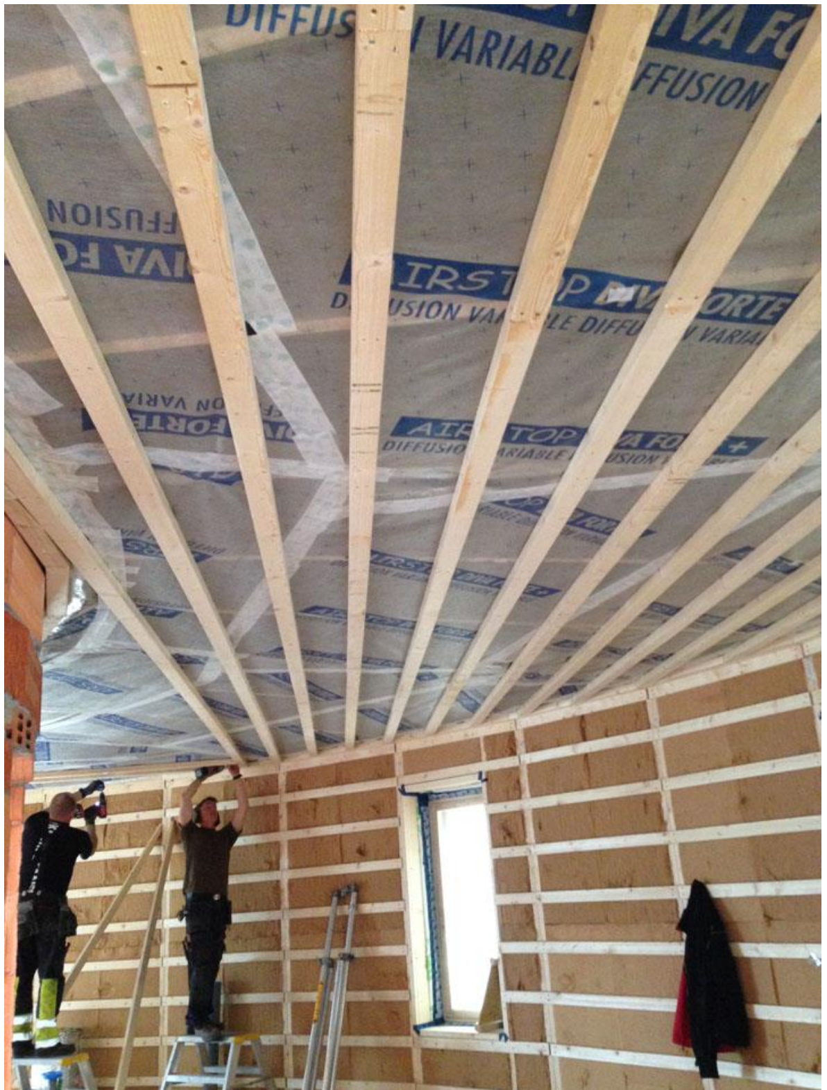
Figure 9. Installation of air barrier for ceiling, all seams properly taped [31].
