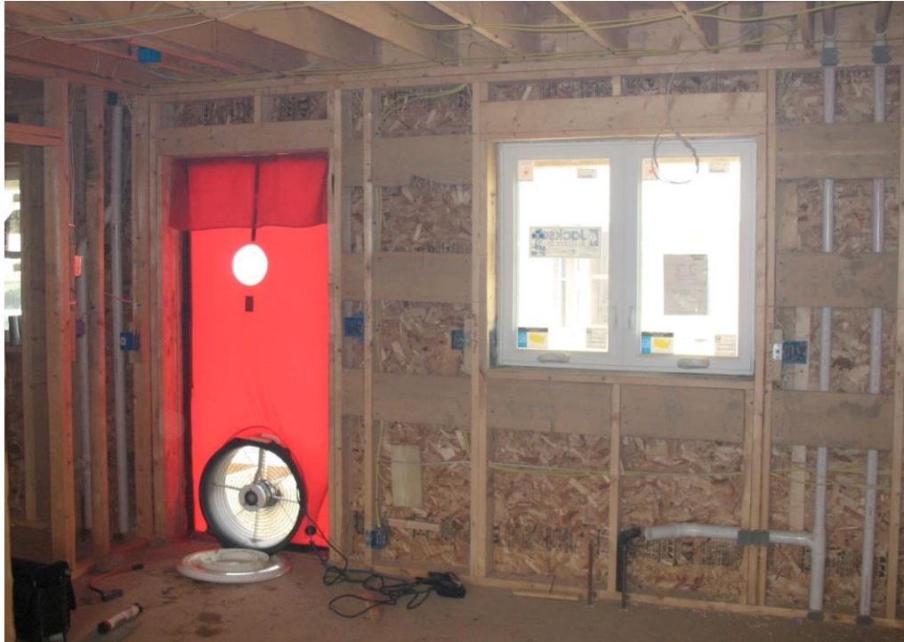
Figure 14. Blower Door Test installation [28].
