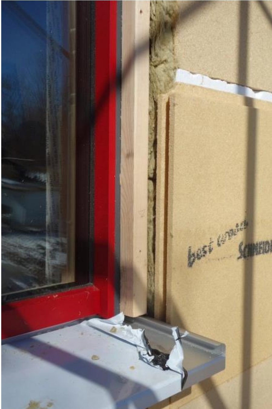
Figure 11. Insulation tight at the window frame [43].
