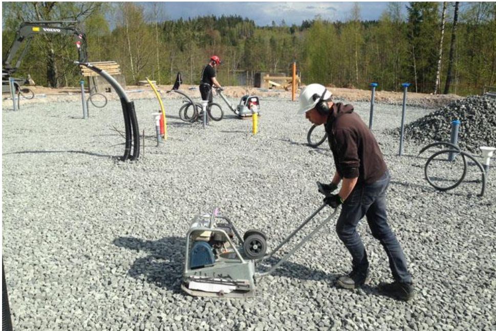
Figure 1. 300 mm of macadam for ground work [31].
