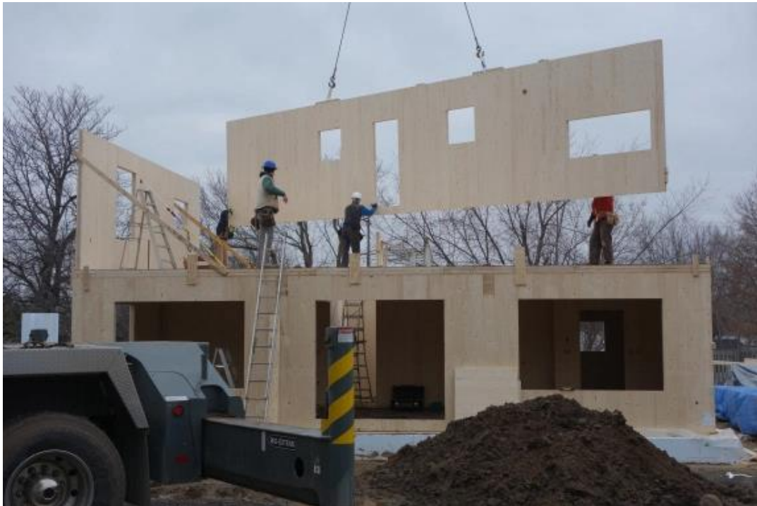
Figure 5. Second floor wall being craned for assembling [41].
