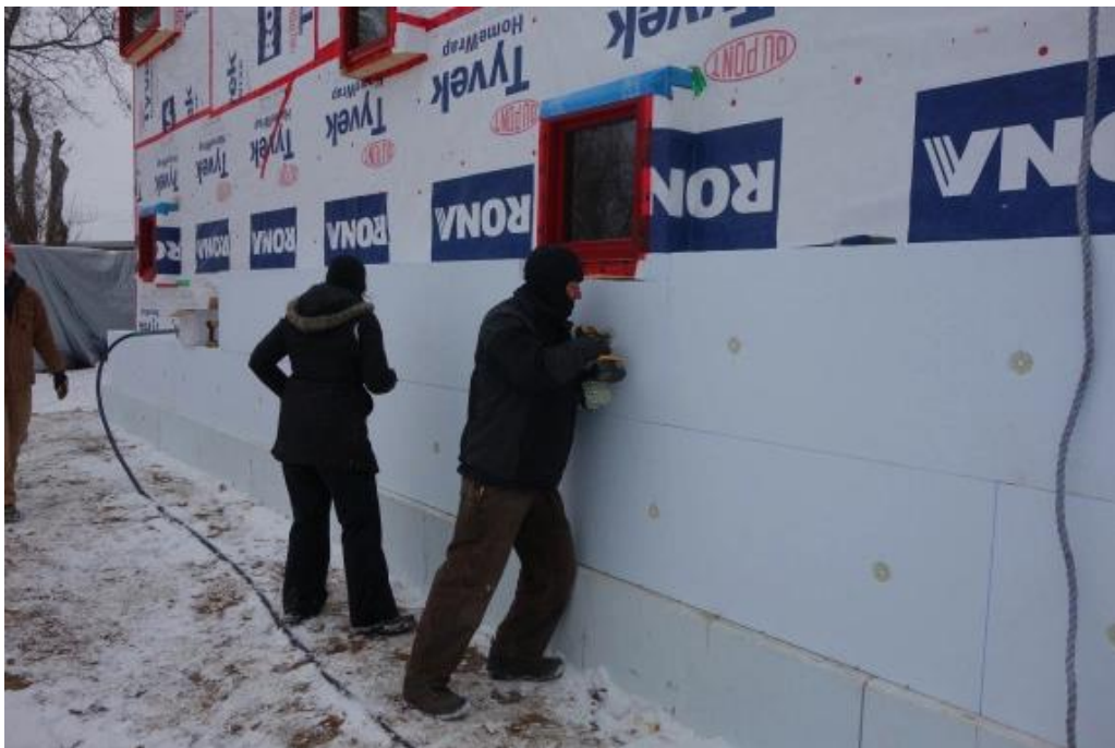
Figure 6. Two base EPS type II layers for wall insulations [36].
