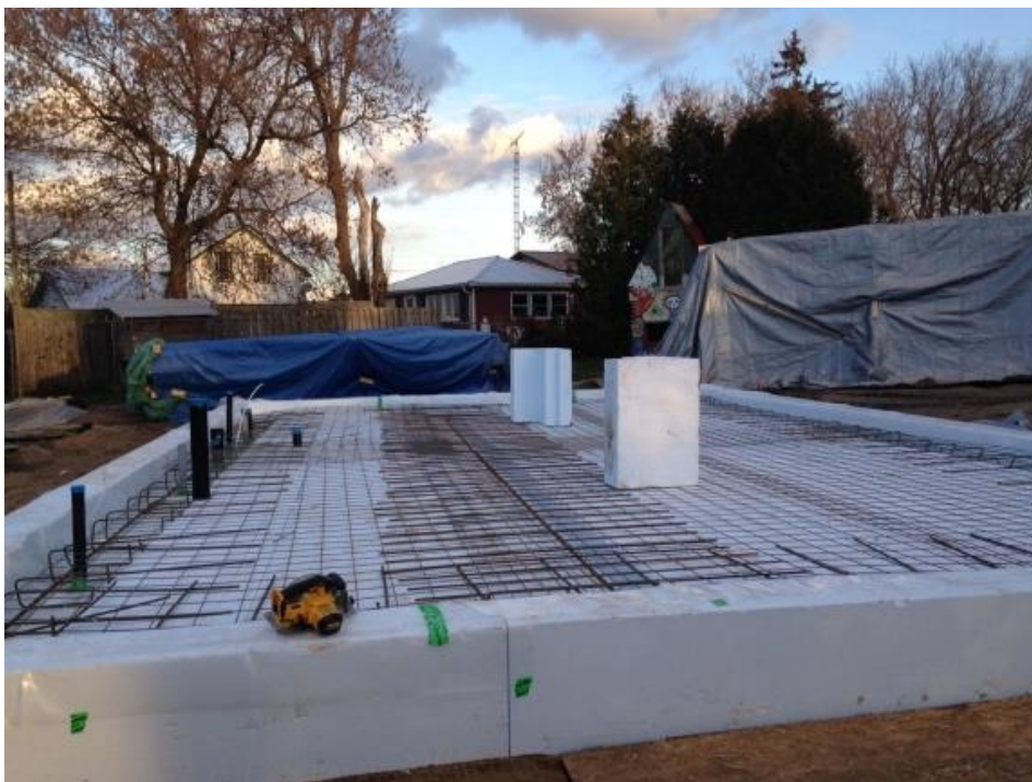
Figure 4. Reinforcement for base floor concrete slab on 300mm EPS [40].
