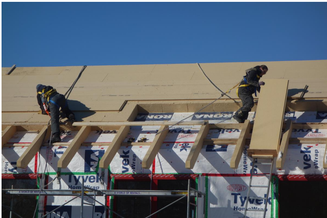
Figure 8. Installation of roof insulations, fiber panels [42].
