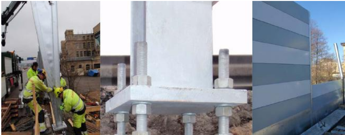
Figure 2.4 Views of the structure
