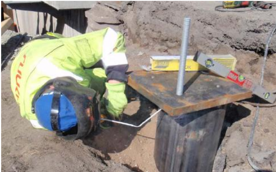
Figure 2.3 Installation of base plate by welding
