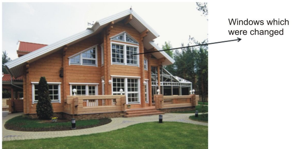
Figure 4.1 Windows of the house which were changed
