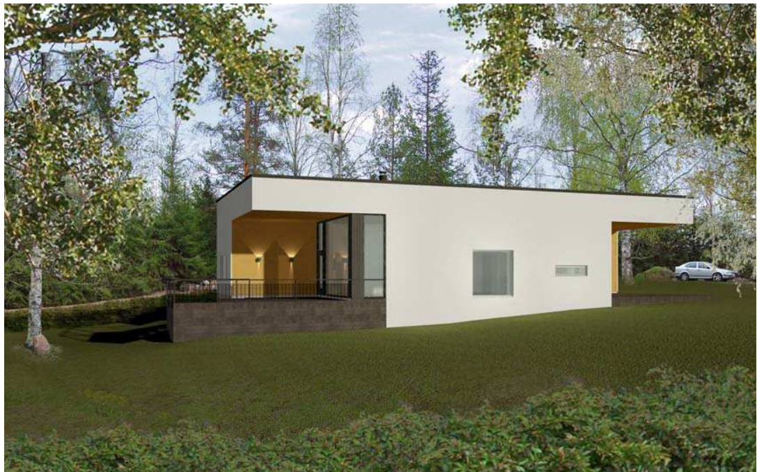
Figure 3.3 Multi-Comfort pilot project in Nummela, Southern Finland (Lylykangas, K. 2009)
