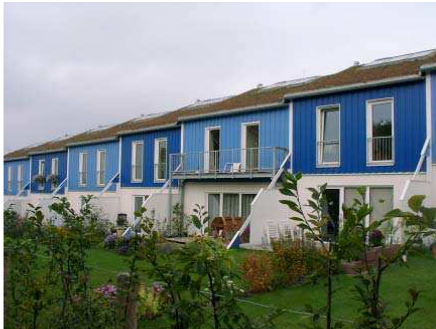
Figure 3.1 Passive Houses in Kronsberg, Hannover (Feist 2001)
