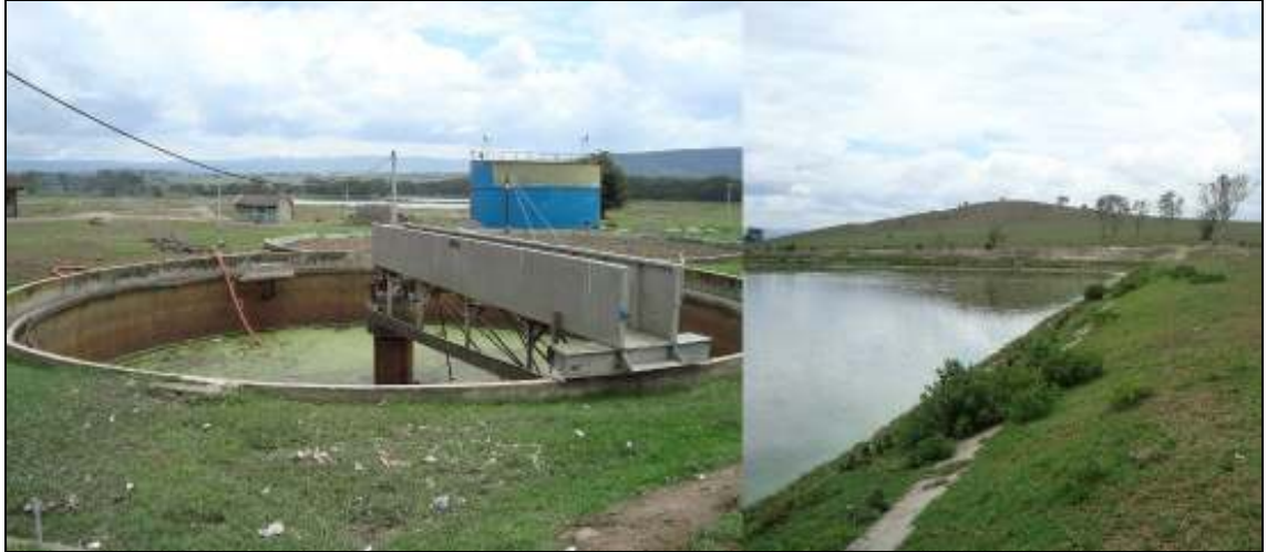
Picture 8: Town Sewage Treatment Installation on the east side of the town was commissioned in 1956 and has a capacity of 6600m 3 /day (State of Environment Report 2009, 18, 23) (Photo: Nurmi L. 2009)
