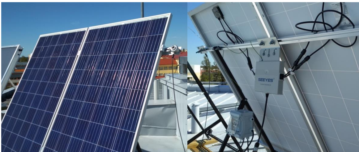
Figure 25. Photovoltaic system assembled on the roof.
