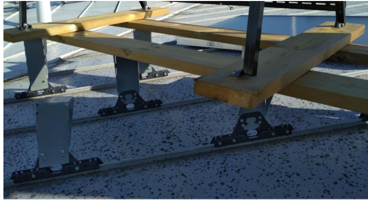
Figure 28. Basement of the structure for the photovoltaic system.
