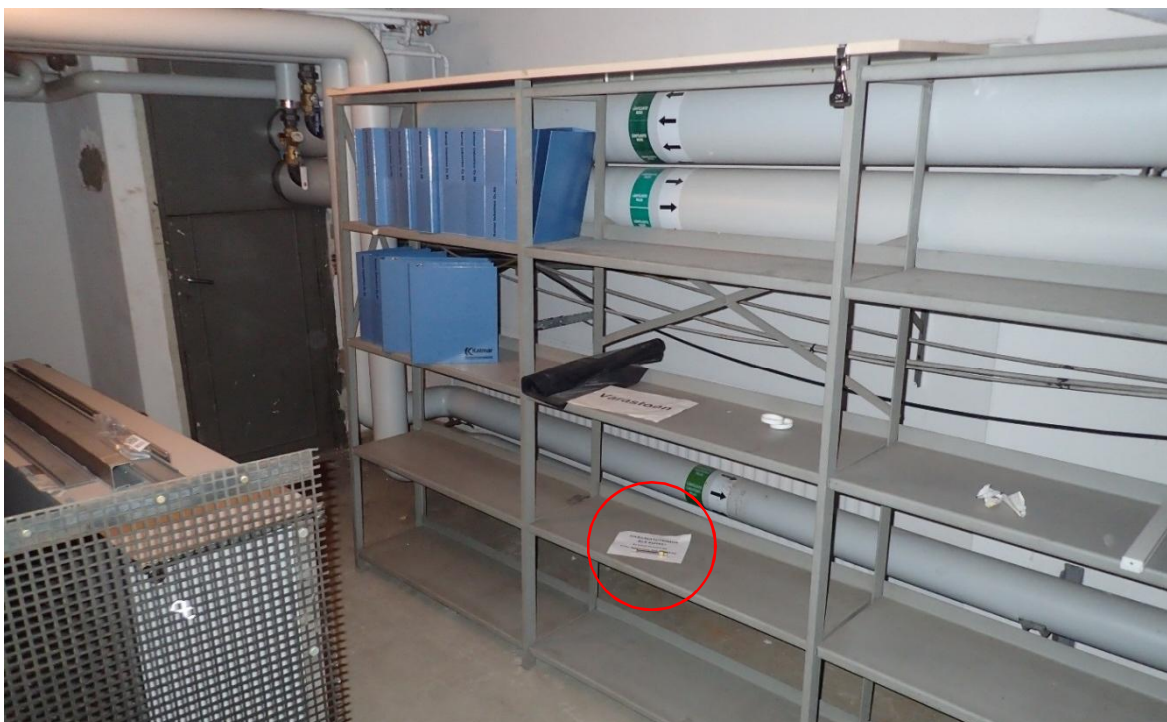
PICTURE 11. Indoor air sampling point SI2 in the administration building (Ramboll/Parviainen, 28 July 2016)
