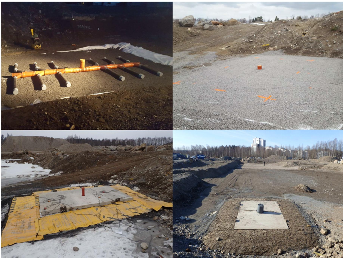
PICTURE 7. Photos of a soil gas venting test structure where a concrete slab with sub-slab ventilation was placed near groundwater table (Ramboll/Parviainen 2016)
