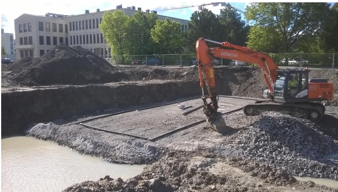
PICTURE 8. A photo taken during the installation of the horizontal soil gas test setting no 1 (Ramboll/Sillanpää, 28 June 2017)
