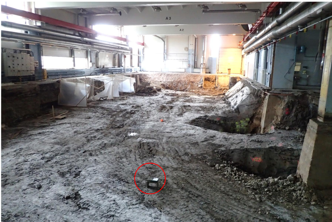
PICTURE 13. Indoor air sampling point SI11 in the open excavation pit inside the old factory. The silty soil under the sampling tube was still highly contaminated. (Ramboll/Parviainen, 28 July 2016)
