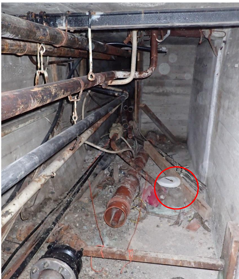
PICTURE 12. Indoor air sampling point SI10 in an old pipe channel (Ramboll/Parviainen, 28 July 2016)
