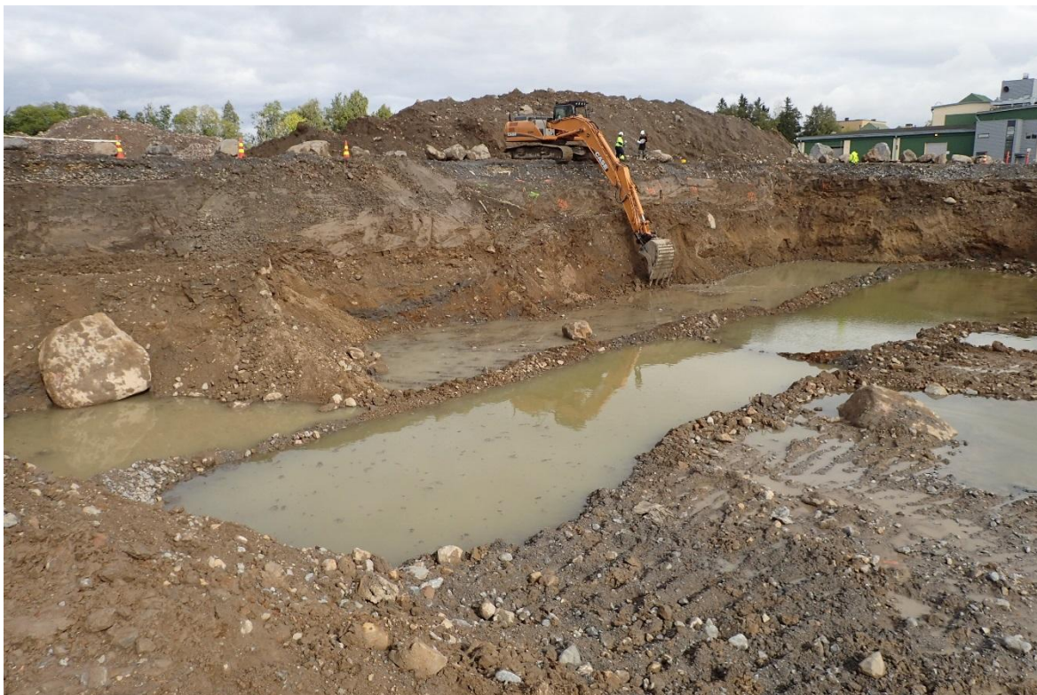
PICTURE 3. In many parts of the area the contaminated soil was excavated until below the groundwater table and delivered for further processing at external reception sites specialised in contaminated soil treatment (Ramboll/Parviainen, 7 Sep 2015)
