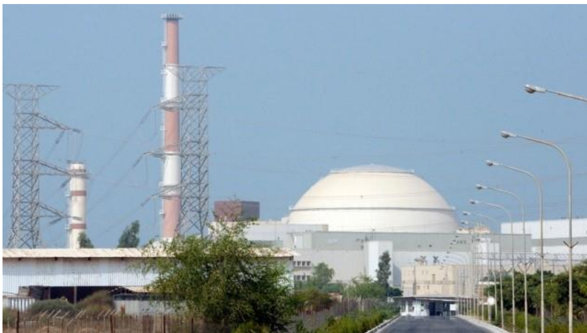
Figure 5 Completed Bushehr NPP in Iran
