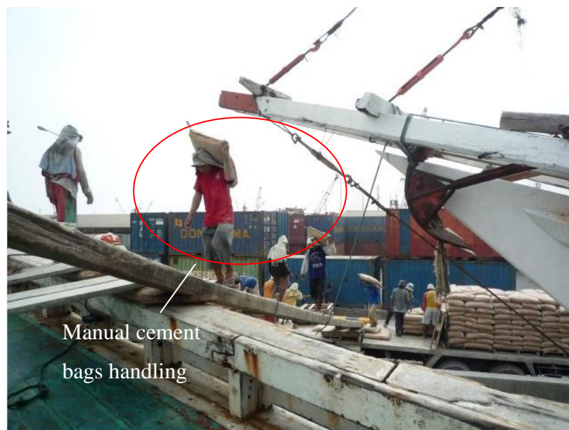
FIGURE 23. Cement bags loaded with manpower (CEL Consulting, picture library, Indonesia, May 10 2010)
