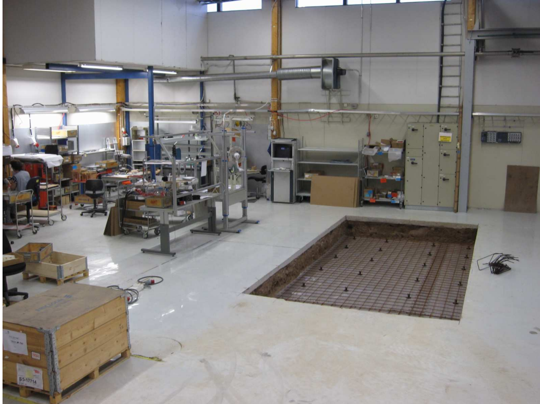
Figure 19. Floor is opened and rebarred for concrete footing.
