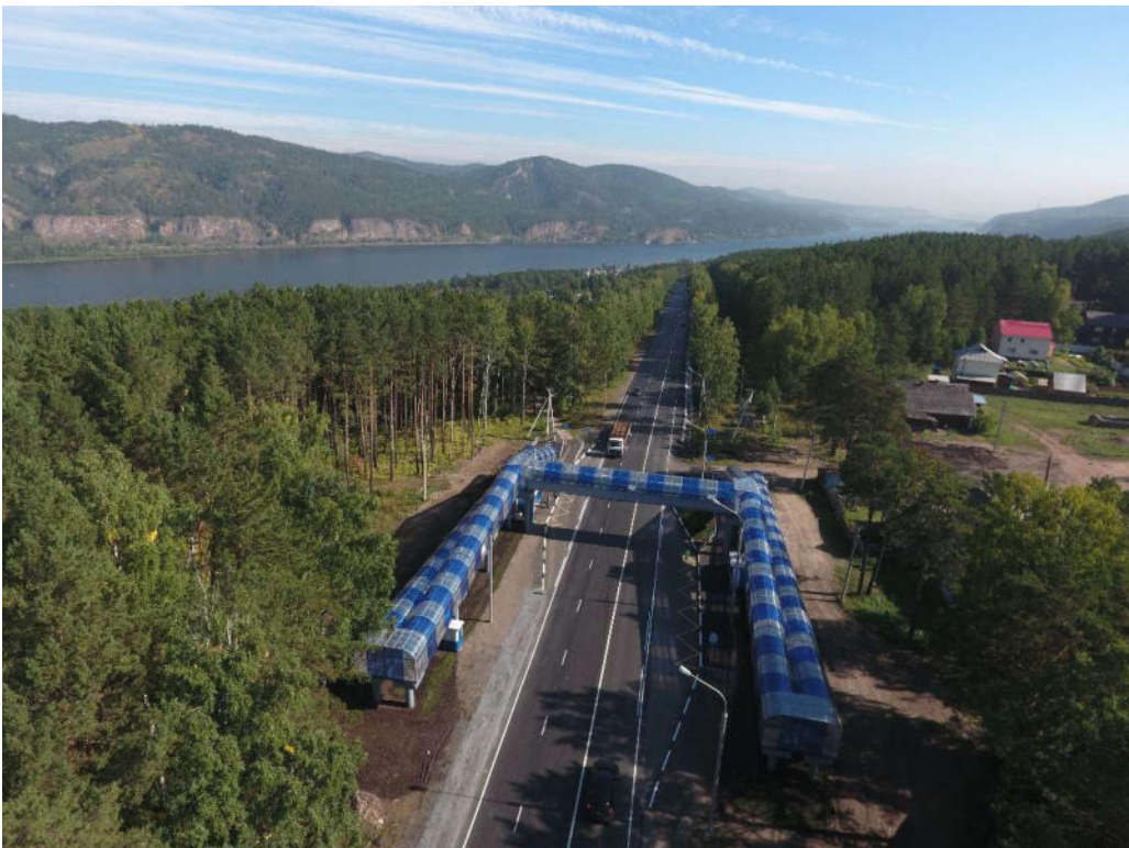
Figure 8.8 Typical pedestrian overpass crossing at the highway with long ramps (image from rosavtodor.ru)
