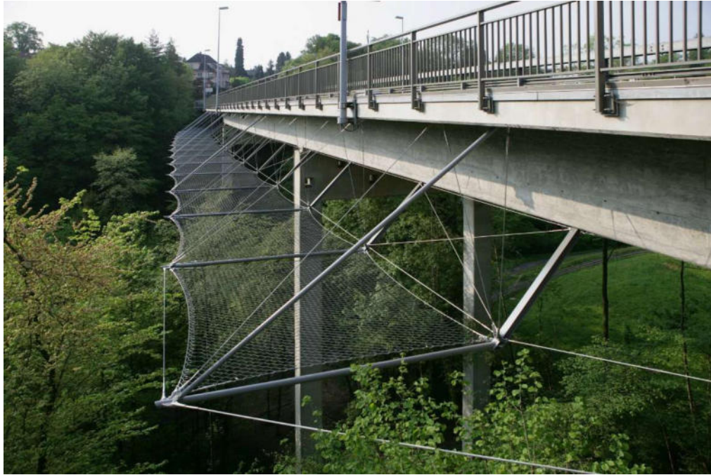
Figure 4.2 Prevention net at the bridge (image from jakob.com)
