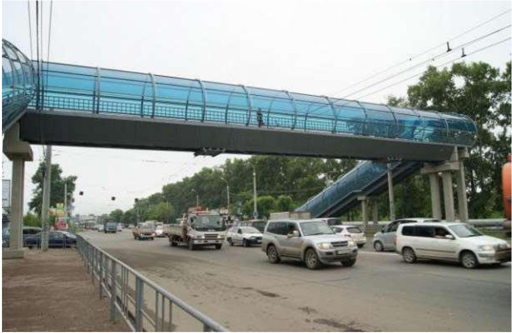
Figure 8.7 Typical pedestrian overpass crossing at the wide street in the urban area (image from news.rambler.com)
