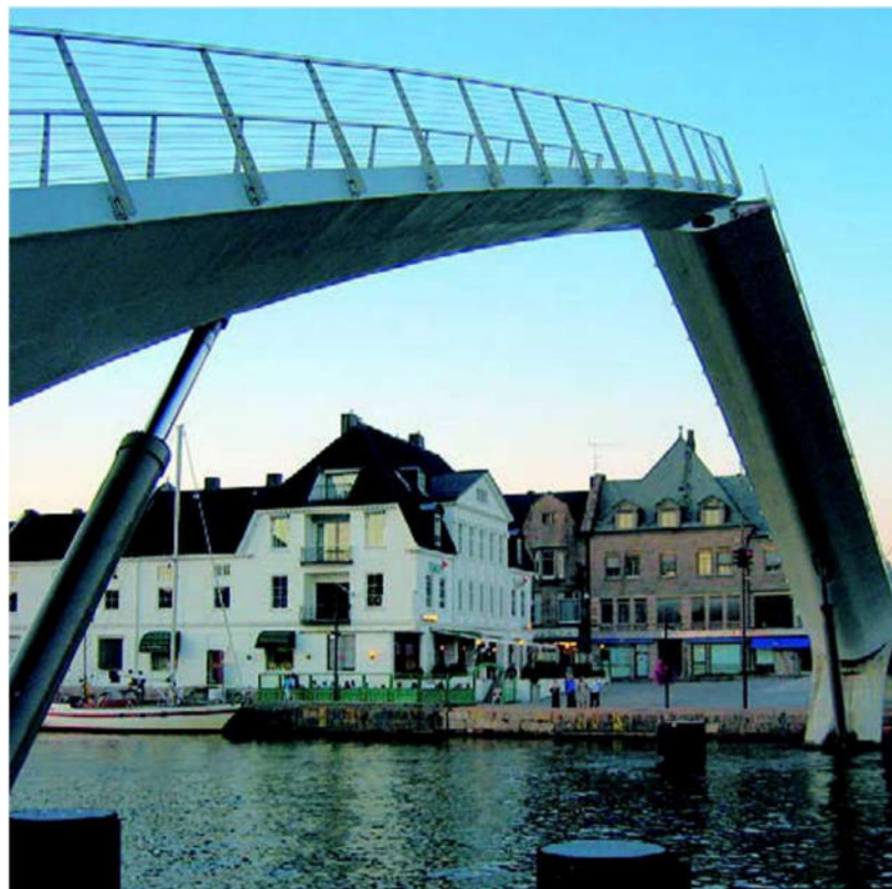
Figure 3.6 Bridge in Fredrikstad made from CRP (image from Keil 2013, p.86)
