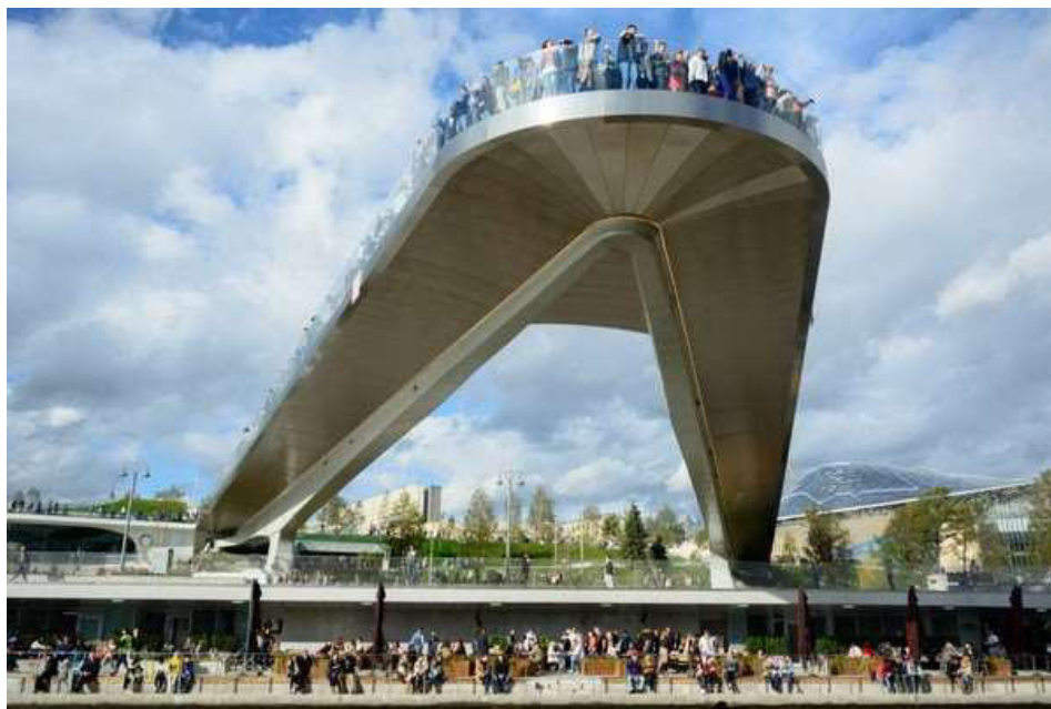
Figure 2.11 Cantiliver Bridge in Zaryadye Park (image from mos-holidays.ru)
