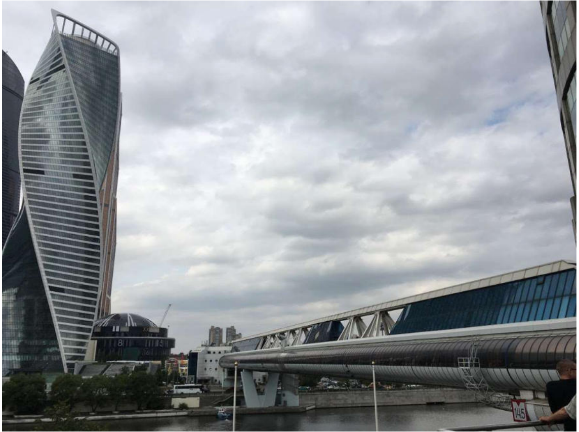
Figure 2.15 View of the Bagration Bridge (photo by the author)
