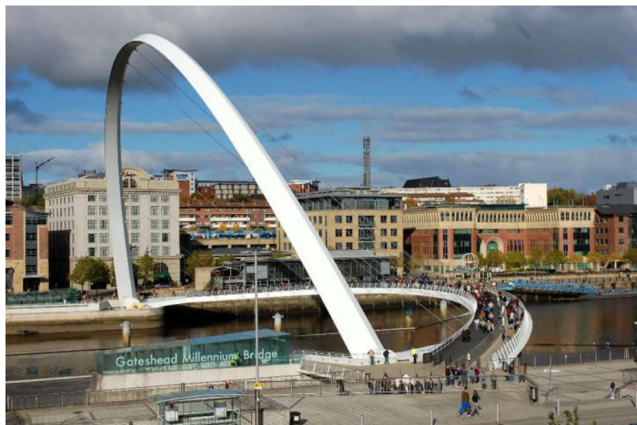
Figure 2.21 View of the Gateshead Milleium Bridge from the Tyne embankment (image from traveltriangle.com)
