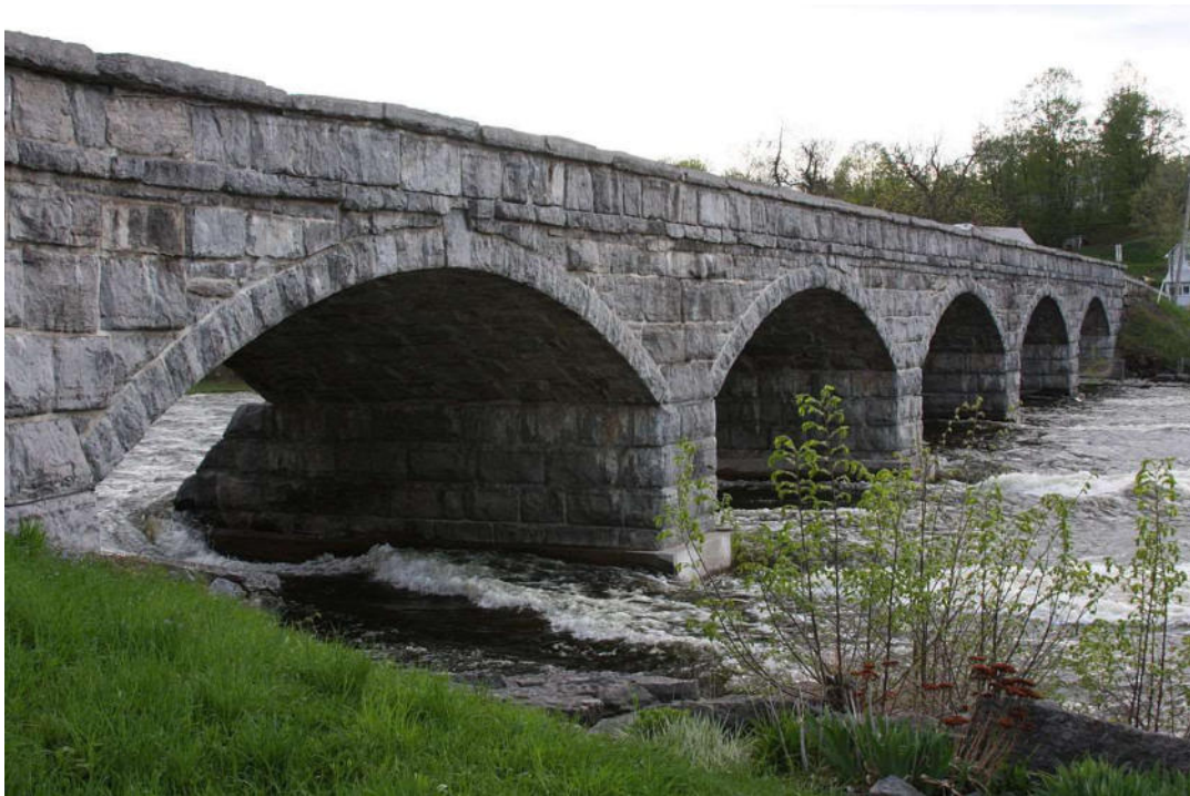
Figure 3.11 Stone bridge at Pakenham (image from Wikipedia)
