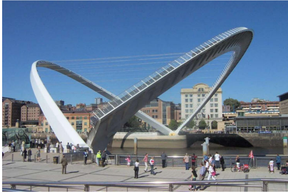
Figure 2.19 Gateshead Millenium Bridge in the tilted position (Wikipedia)
