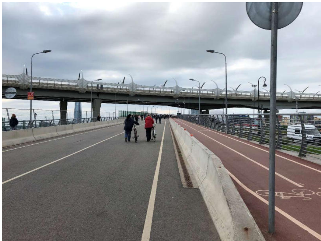
Figure 8.3 Planning of the span of Yahtenniy Bridge (photo by the author)
