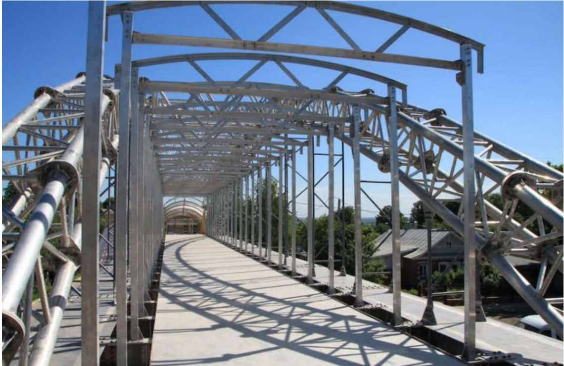
Figure 3.3 Aluminum bridge (image from aluminiuminsider.com)
