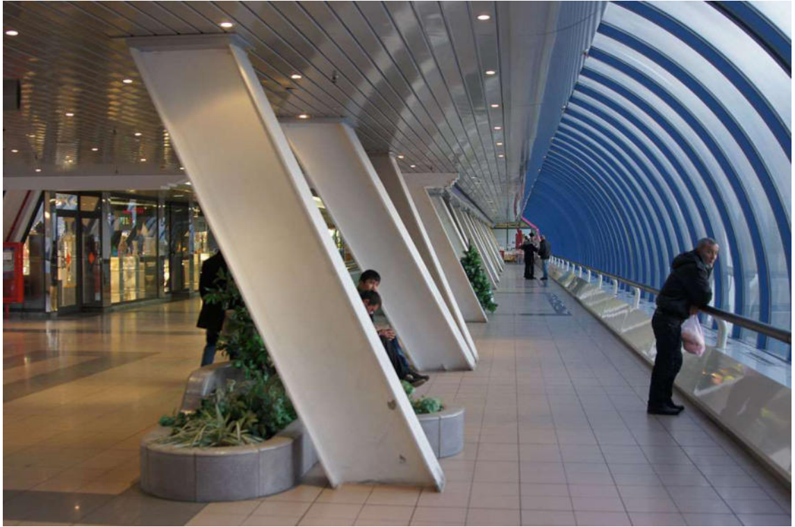
Figure 2.16 View of the Bagration Bridge from the inside (image from travel.wmouse.ru )
