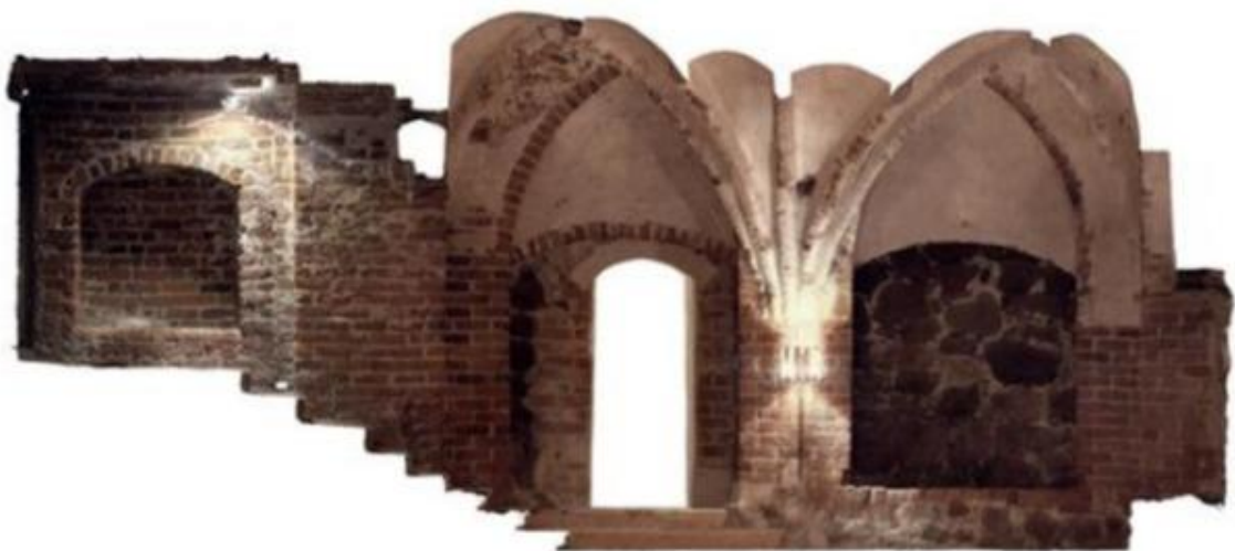
Figure 3. Excerpt of a laser scanning point cloud of a historic building (Common BIM Requirements 2012. Series 2: Modeling of the starting situation, 2012).
