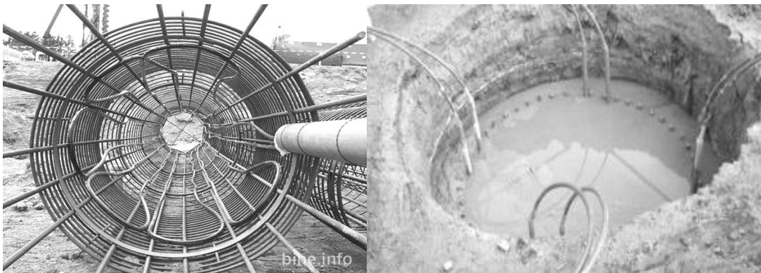
FIGURE 11. Pile-foundation heat exchanger (BINE informationsdienst, 2010)
