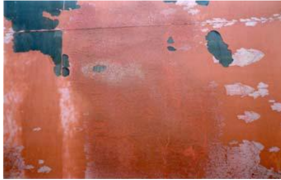
Figure 4. Detachment in coating increase the hull friction 5
