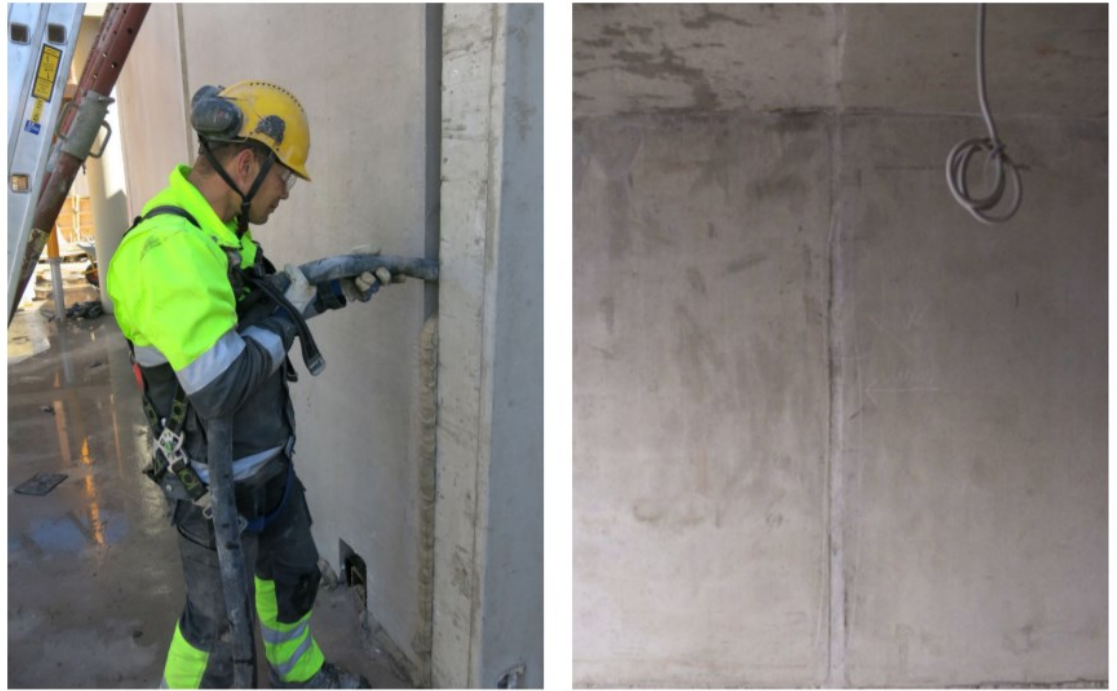
Figure 55 Casting of the joint (Peikko, 2019, p. 27)
