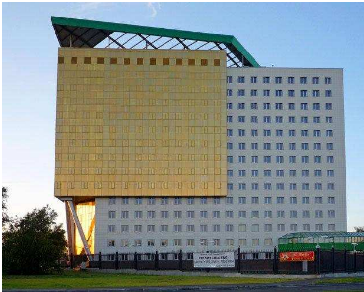
Figure 1.1 Police building of western administrative district of Moscow equipped with R65-BP system.
