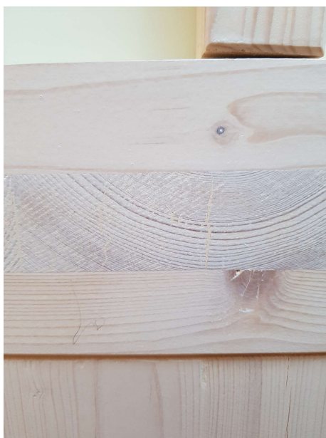
Figur 1. CLT – Cross Laminated Timber.
