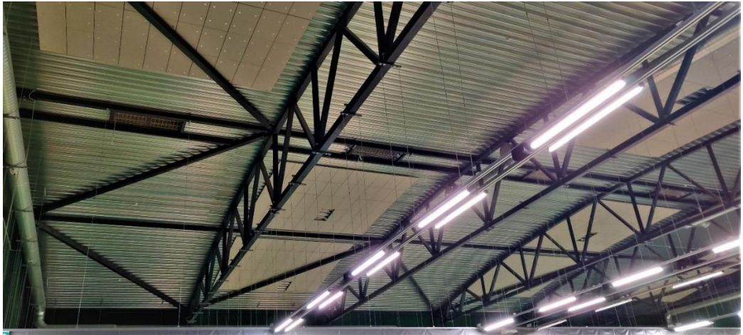
Figure 2. Roof structure of one sport center in Helsinki.
